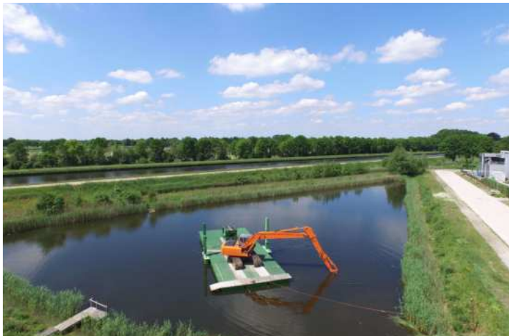
Ponton set with an excavator
